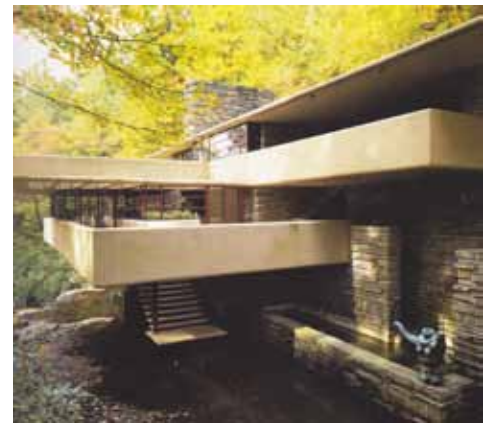
Frank Lloyd Wright. Villa Fallingwater
